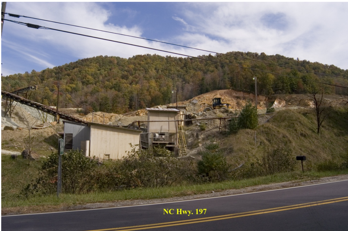
South side of olivine processing plant. Open pit is in background.
