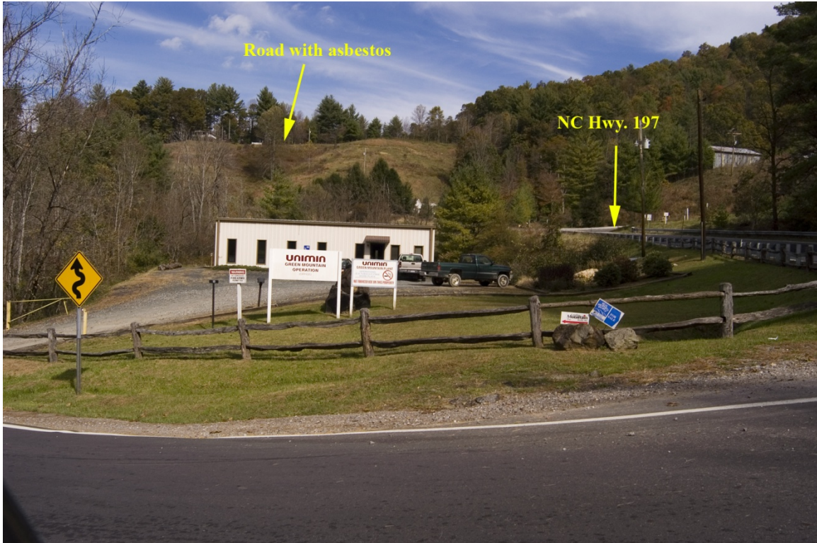
The hill north of the mine office was once the site of a pit or quarry (1984 Burnsville 7.5' Topo).
